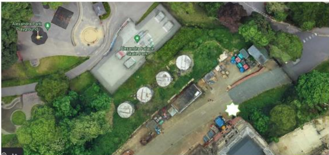
North Service Yard – ANPR camera location
